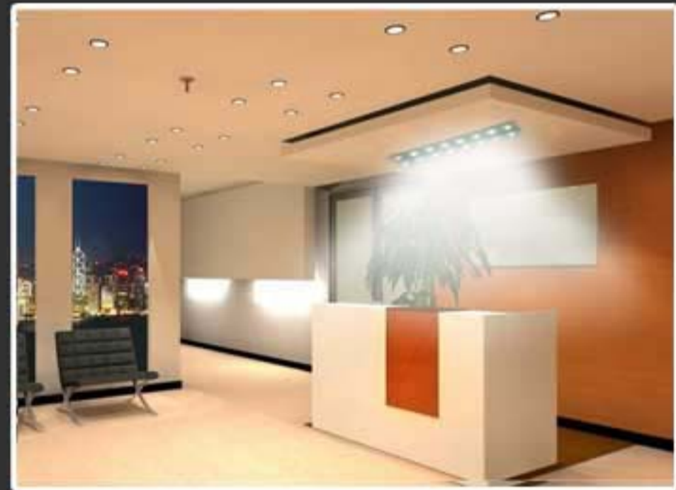
Latest LED based fixtures.
